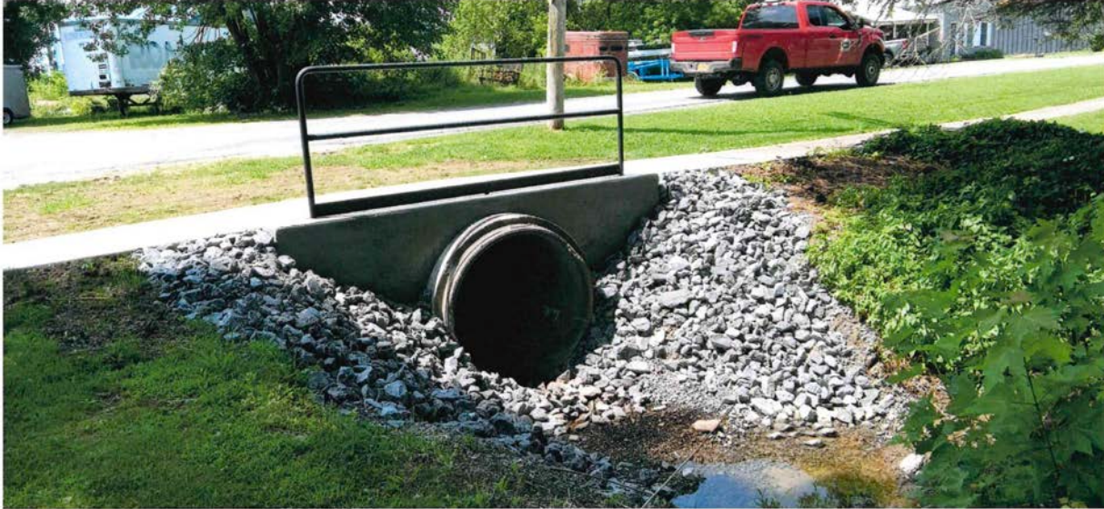
Washington Street Bridge Project
