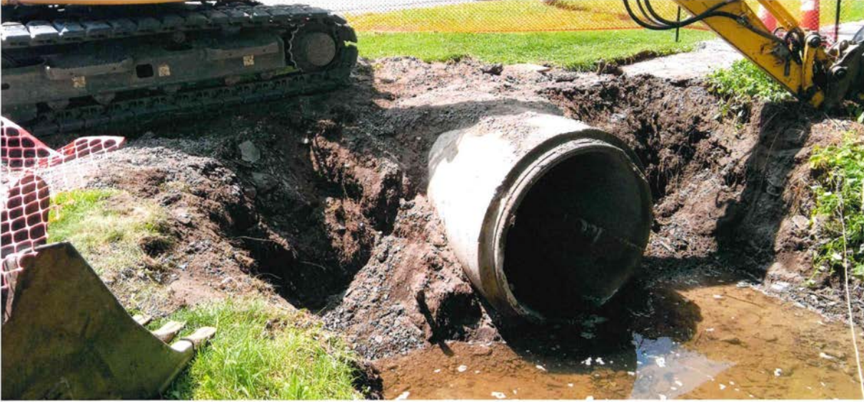
Washington Street Bridge Project
