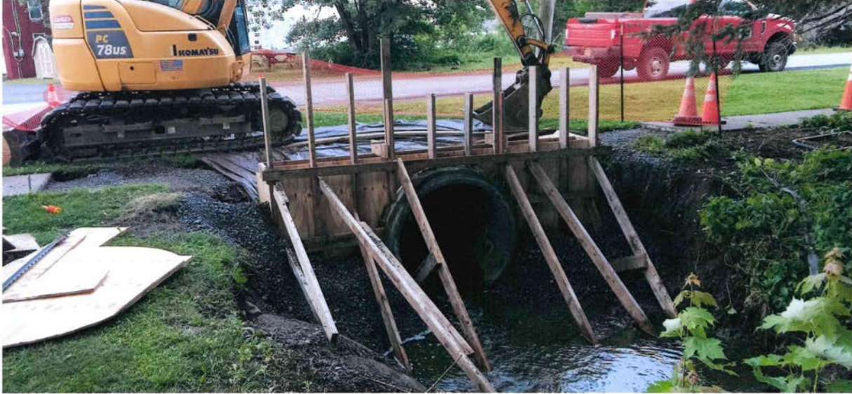
Washington Street Bridge Project
