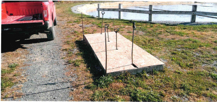
S.T.P. Main Flow Control Chamber Covered
