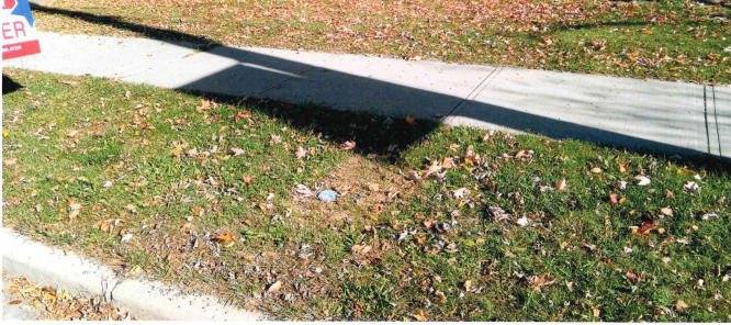
Curb Stop Required 16015 St 12, Vincent
