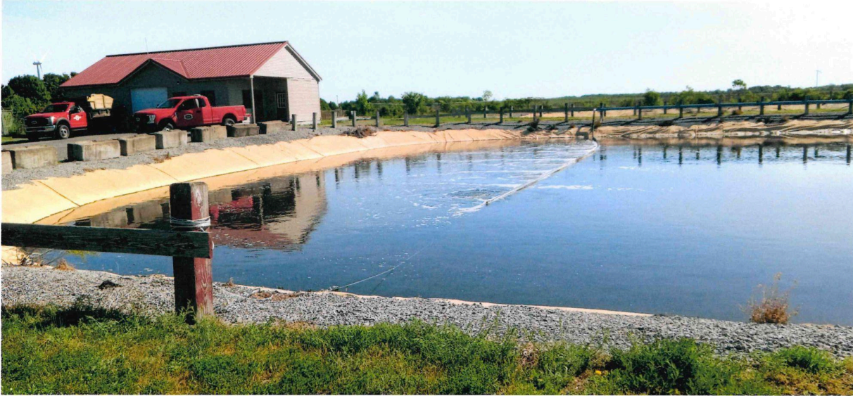
6-9-2026 Repaired broke cable on diffuser line
