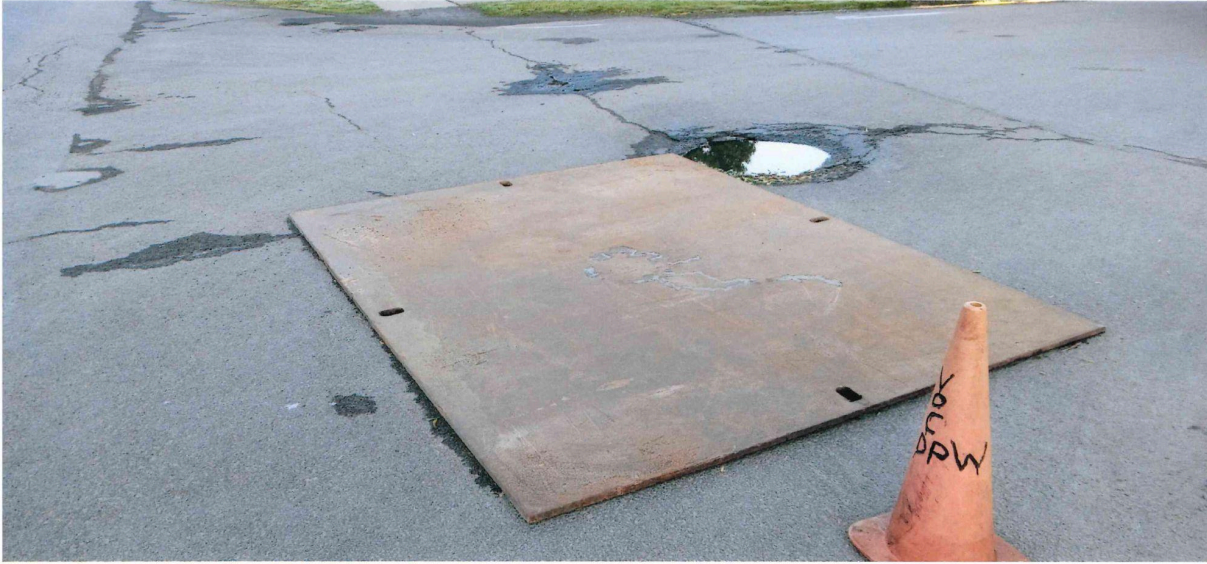
Temporary Fix to Storm Drain on Loud Street
