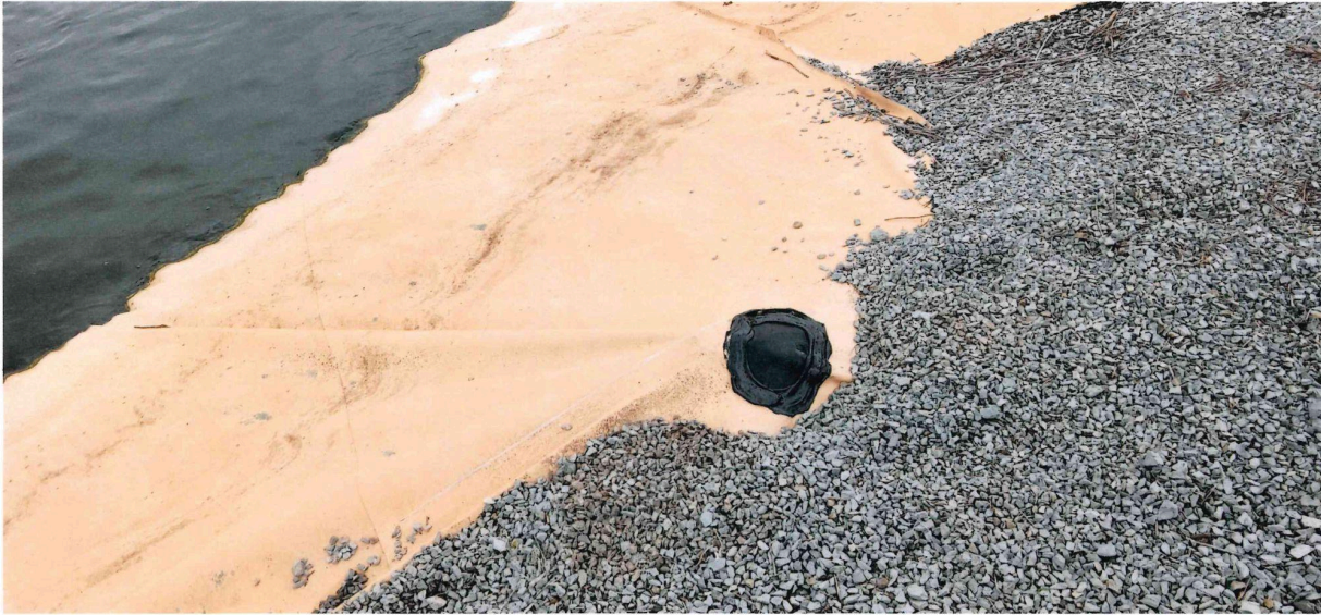
Another Hole Repaired on Shore Line of Lagoon 1 July 28, 2025
